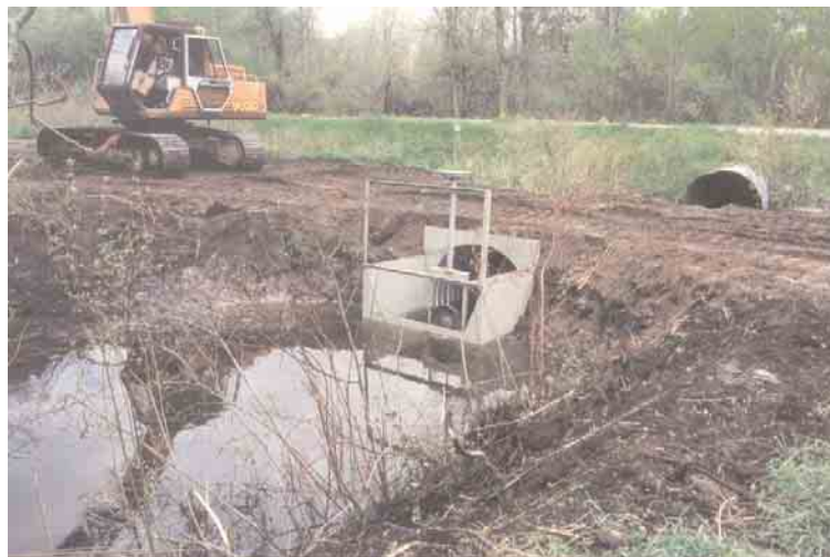
Water Control Structure installation by Norfolk County staff.
